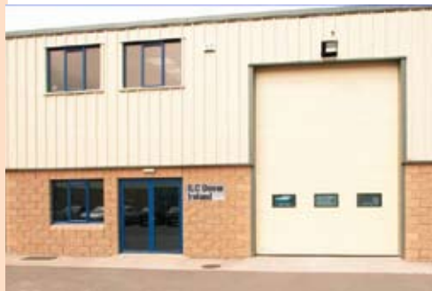
ILC Ireland facility
