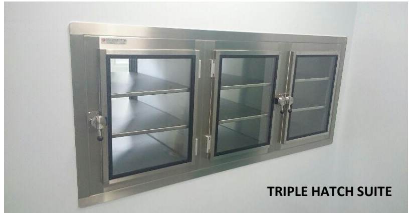
STAINLESS STEEL MECHANICALLY INTERLOCKED TRANSFER HATCH WITH LAMINAR AIR FLOW
