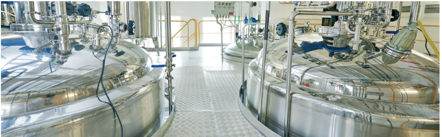
Figure 3: Example of problematic plant areas
